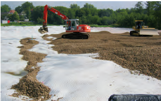
Placement of min. 200mm aggregate
