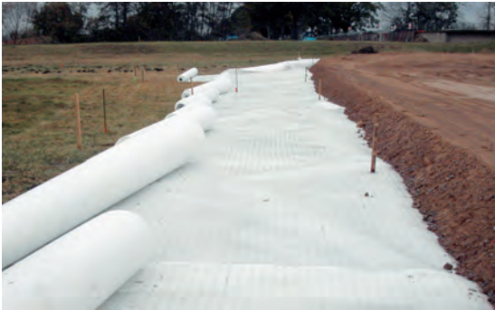
Installed Combigrid® with overlaps
