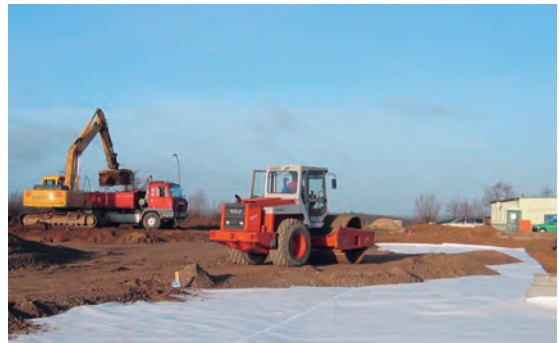
Soil compaction over Combigrid®
