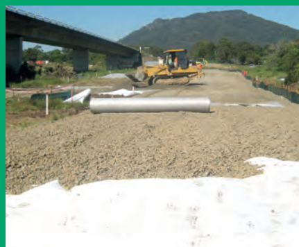
Figure 4 Combigrig® unrolled and covered with topsoil
